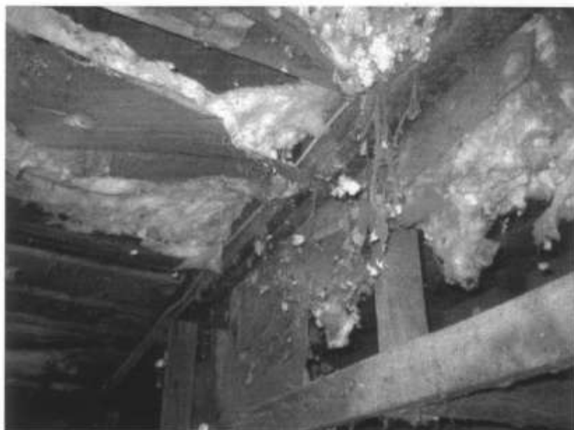
The garage in which the ferrets were housed was heavily damaged by mice. Above, insulation, filled with mouse feces, hung loosely from the ceiling.
